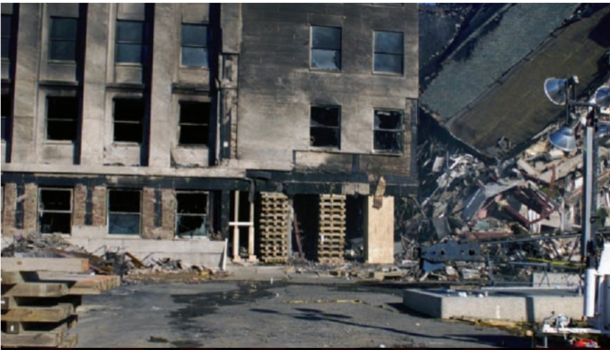
Shoring up the E-Ring
